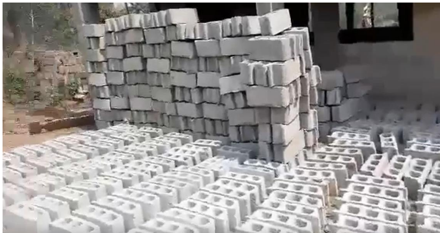
The newly made bricks ready for the first floor roof (second floor).
