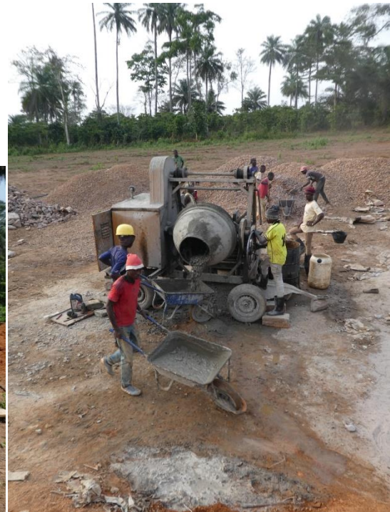
Initially all the cement was mixed by hand. A cement mixer was hired and sped up the work considerably.
