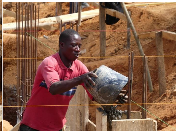
Once the wire framework for the foundation pillars were in place, they were cemented in prior to being framed up and being manually filled with cement.
