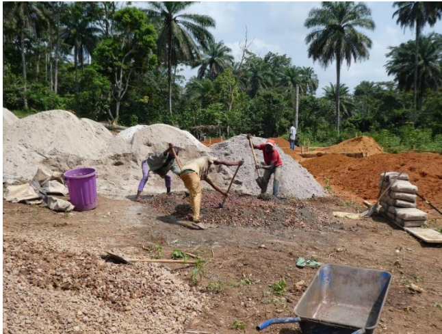
Initially all the cement was mixed by hand. A cement mixer was hired and sped up the work considerably.
