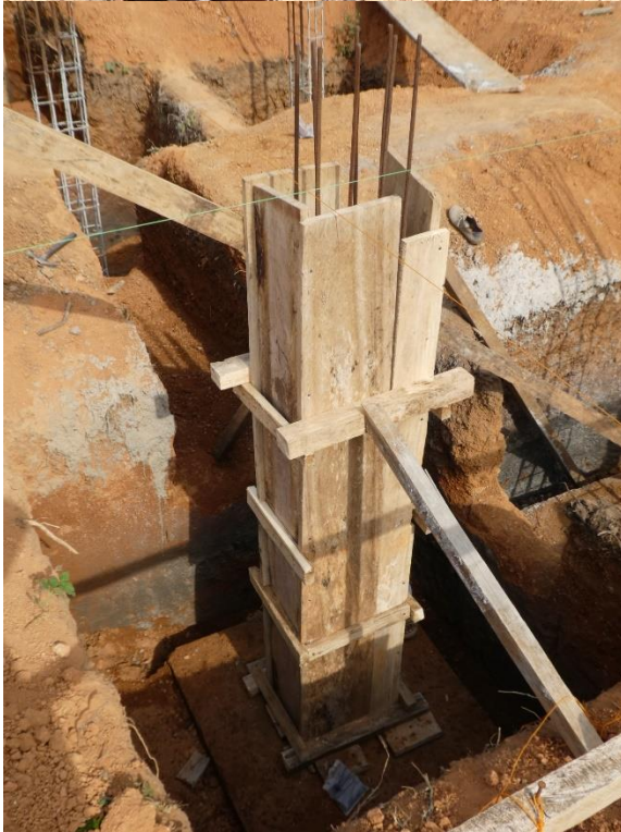
Once the wire framework for the foundation pillars were in place, they were cemented in prior to being framed up and being manually filled with cement.
