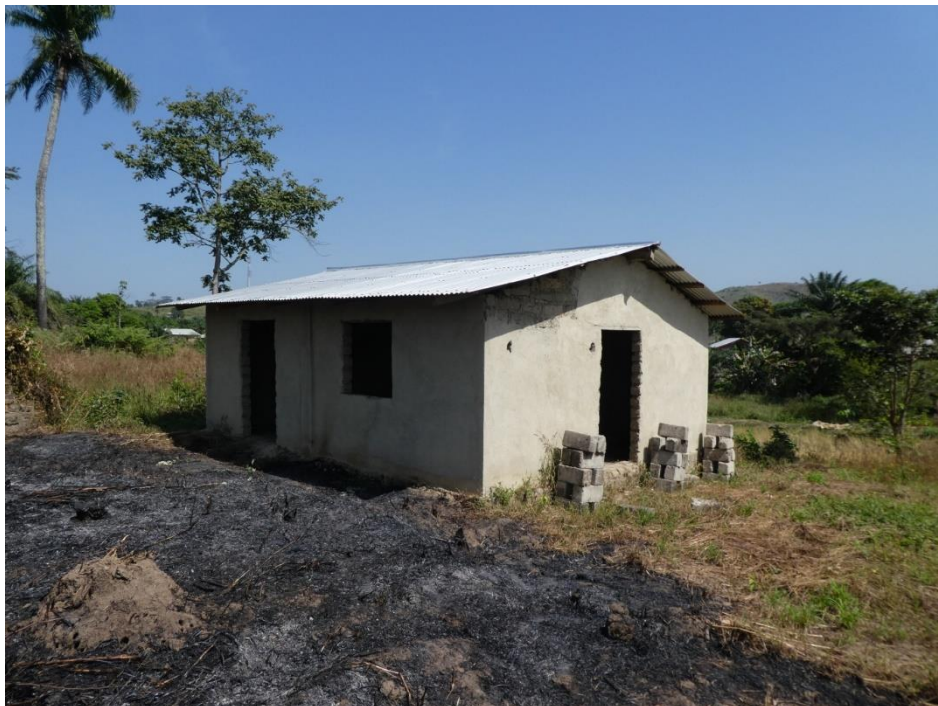
The worship hall being constructed at Macenta.
